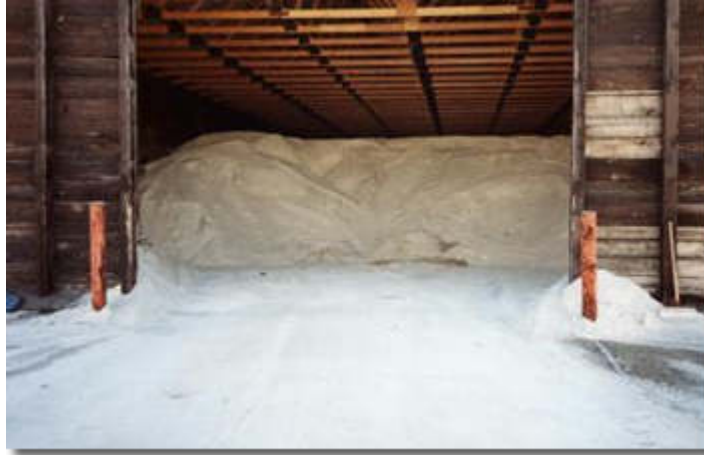
While this salt storage is in a covered area, there is considerable spillage outside.
